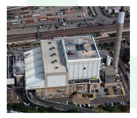
Veolia's South East London Combined Heat & Power (SELCHP) energy recovery facility (ERF) takes collected waste from the surrounding boroughs of London and converts it into electricity and heat through a series of processes.
